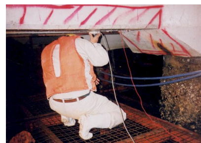
Inspection of chloride induced deterioration of a concrete structure.
